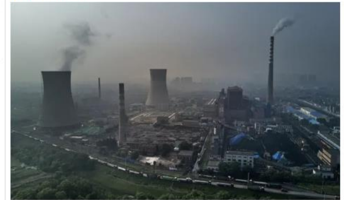
A state-owned coal-fired power plant in Huainan, Anhui province, China. Photograph: Kevin Frayer/Getty Images
