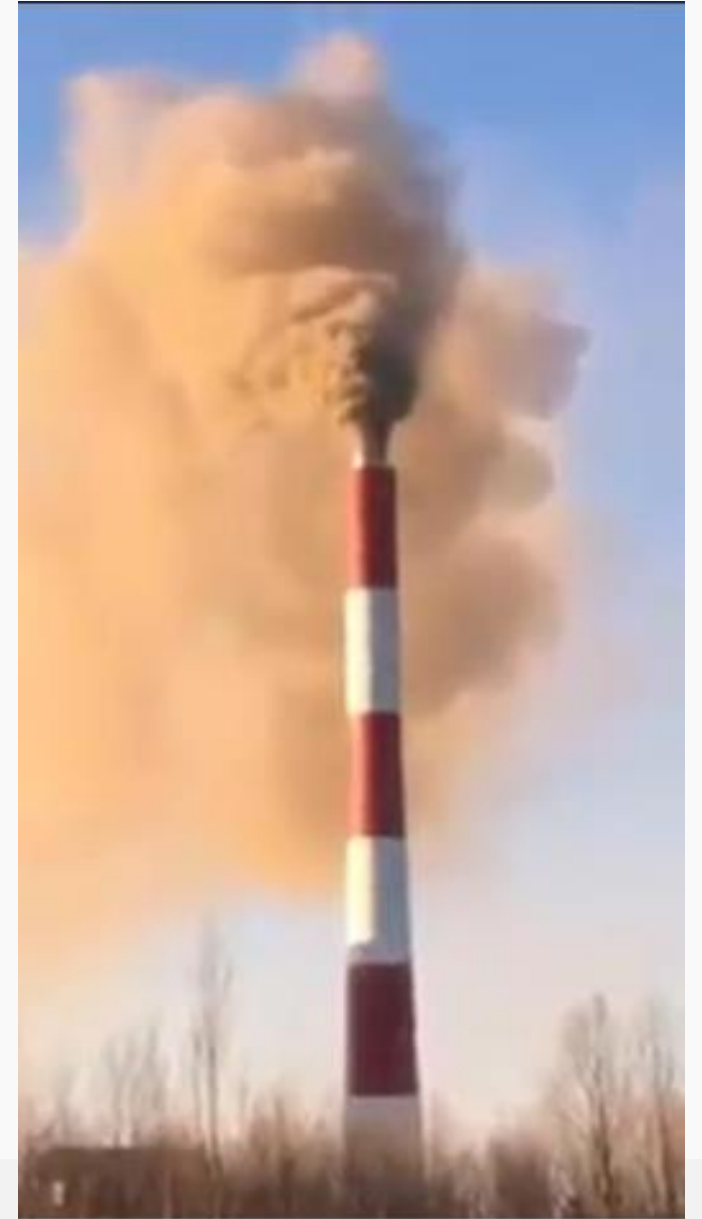
Stanari power plant, January 2018,
